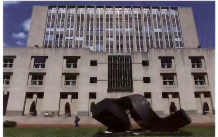
The exterior of Uris Hall
